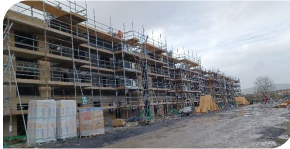
Works ongoing at Robbers Lane, Maugheraboy
