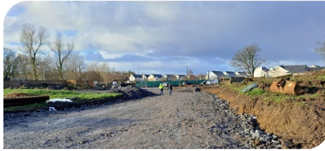
Works commenced on 16-unit scheme at Grange
