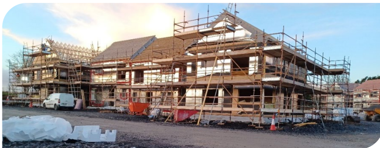
Works underway at Finisklin Sligo
